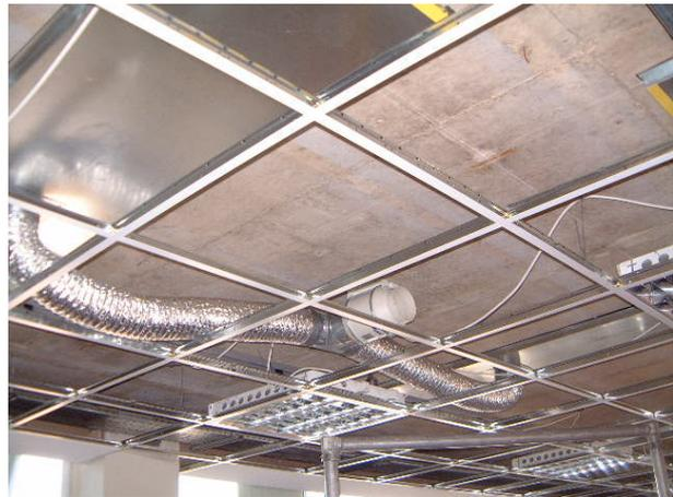
**Figure 11. CoolDeck + PCM installation.**
