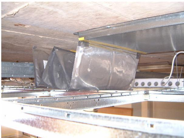
**Figure 10. Installing PCM pouches.**
