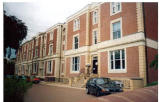
2001: HM Customs & Excise, Wolverhampton – hydrocarbon chiller
